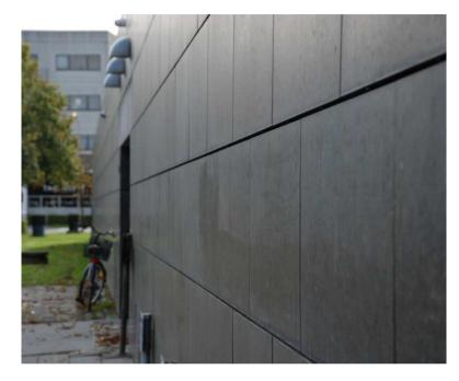
The exterior surface of the library is covered in plates of unhewn Norwegian "Solvåg" stone. These plates have no load bearing function since they are attached merely to the outside of the perimeter wall, only a few centimeters apart, the inner wall consists of limestone.
